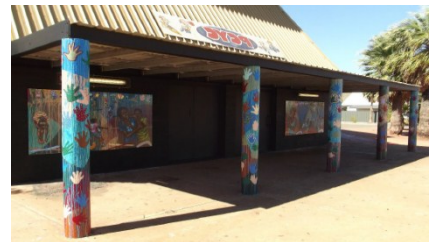
Roebourne Community Hall –after community art project
